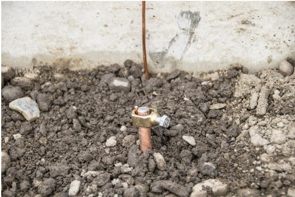
Figure 4.24: Ground wire, connector and 8' (2.5 m) copper plated steel rod. Photo courtesy FGL/IM-PAHO and SELF
