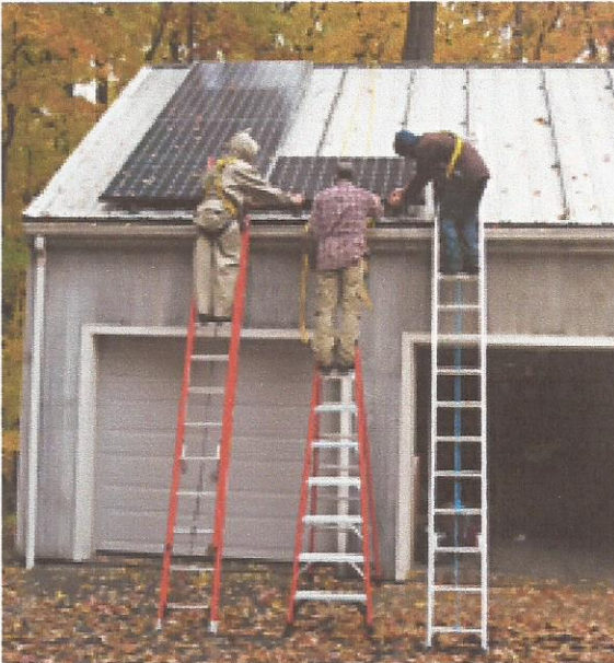
Figure A.2: Use multiple ladders to lift bulky equipment such as PV modules.
