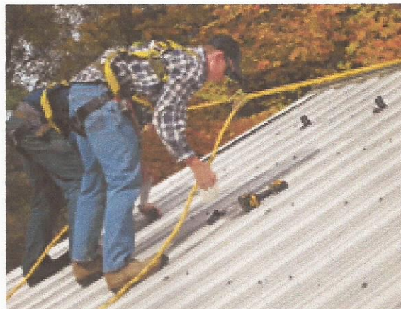
Figure A.7: A worker's lifeline and harness.
